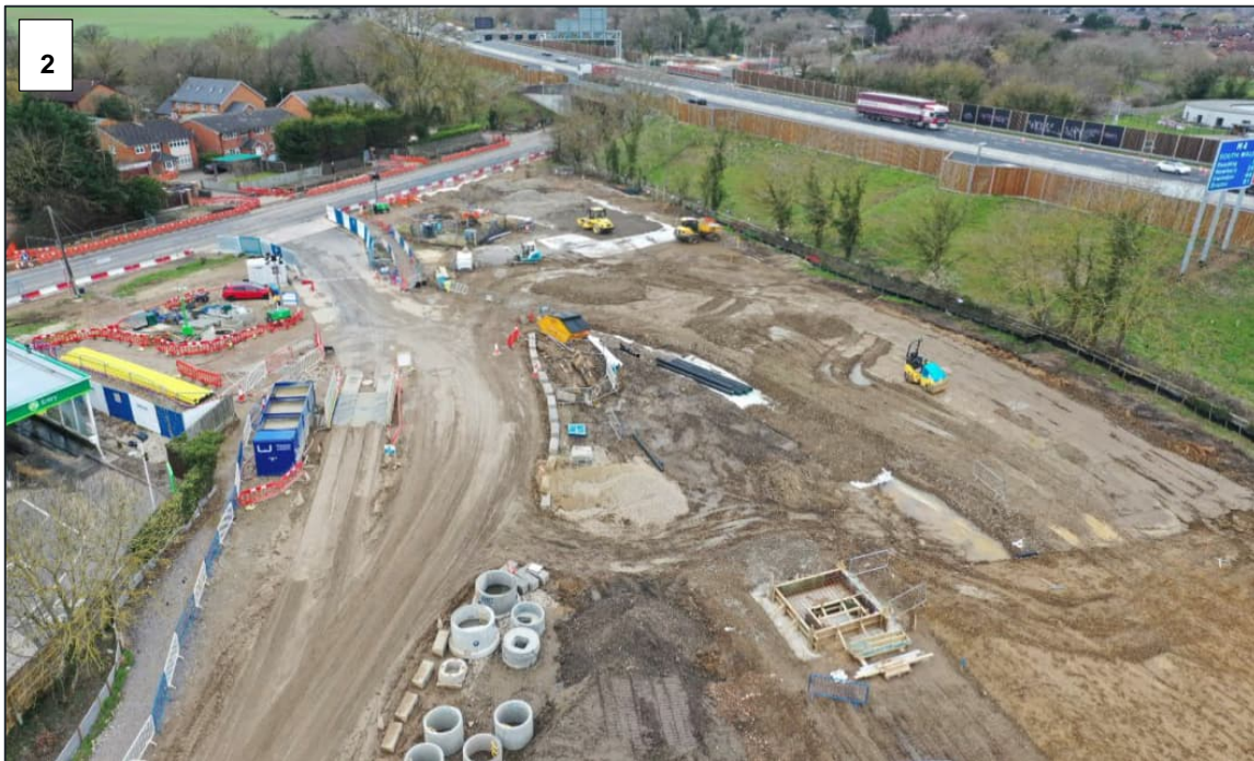
Figure 2-3 - Aerial view of construction of new southern roundabout
