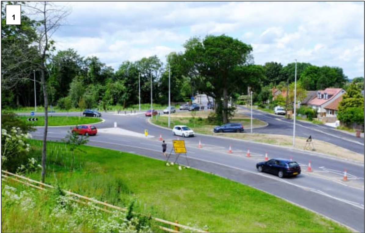
Figure 2-4 - Aerial view of new northern roundabout – now open to traffic
