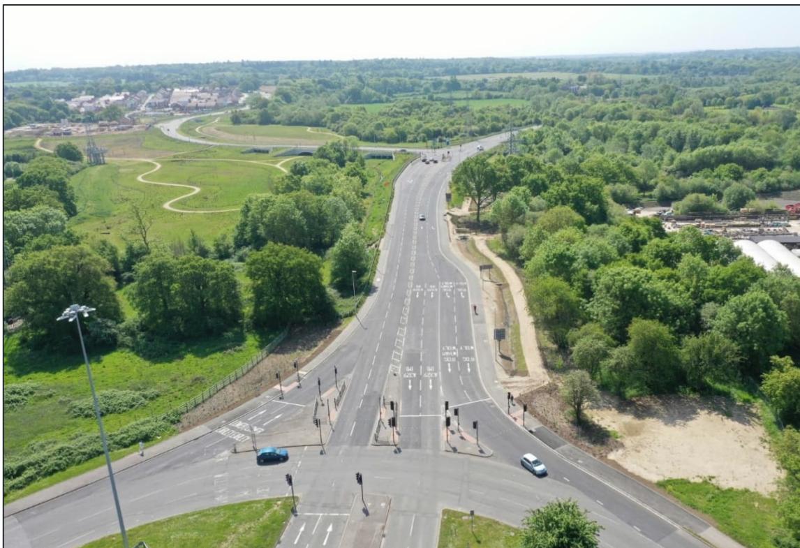
Figure 2-7 - Aerial view of Lower Earley Way Dualling (after)
