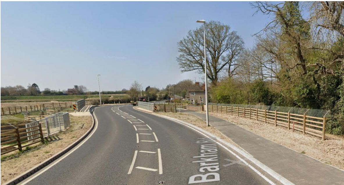
Figure 5-2 - Barkham Bridge - Post construction Westbound approach (Source: Google Images)
