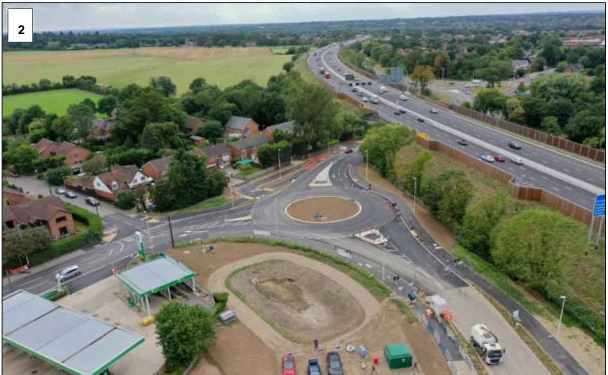
Figure 2-5 - Aerial view of new southern roundabout – now open to traffic
