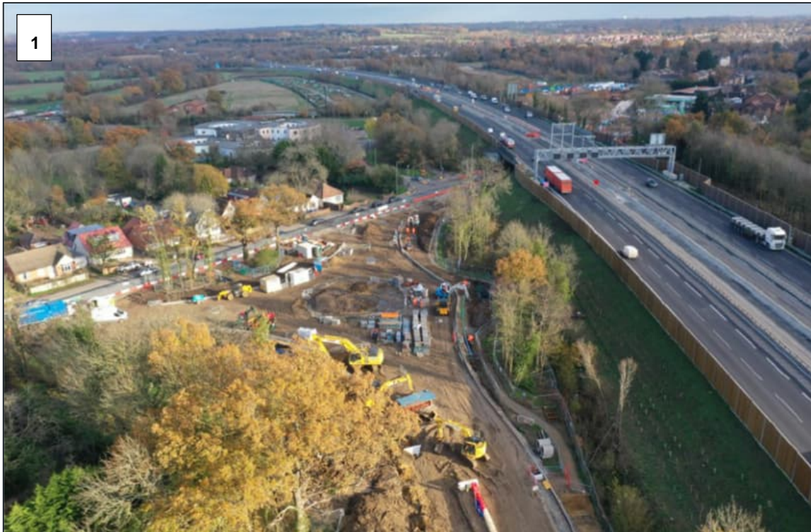
Figure 2-2 - Aerial view of construction of new northern roundabout
